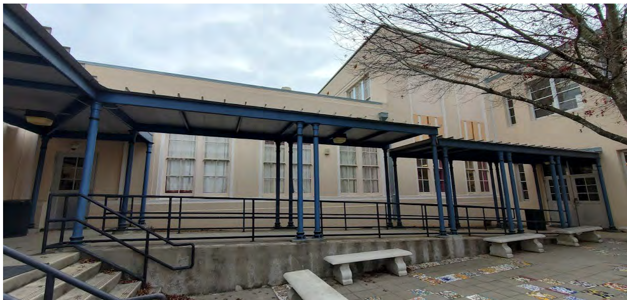
Example of breezeways with metal canopies and columns
